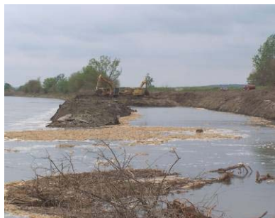
Pilot Channel Under Construction
