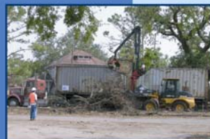
New Orleans Emergency Response Katrina Cleanup Debris removal, demolition
