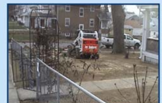
Omaha Lead Site Residential environmental cleanup
